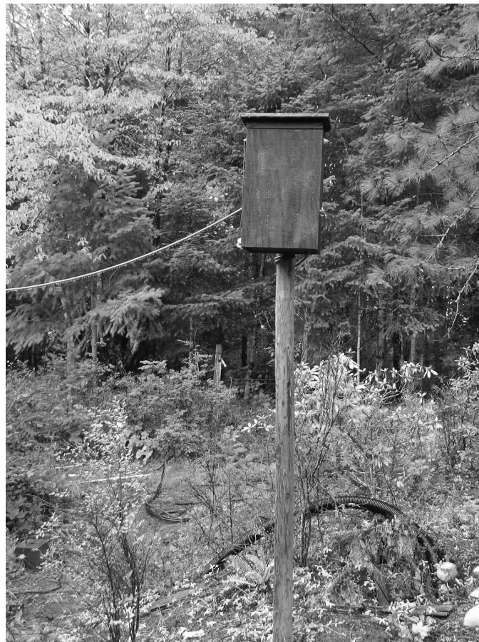
Photo F — The driven element's east leg tuning box. The heavy cable contains the low-voltage control wires.
